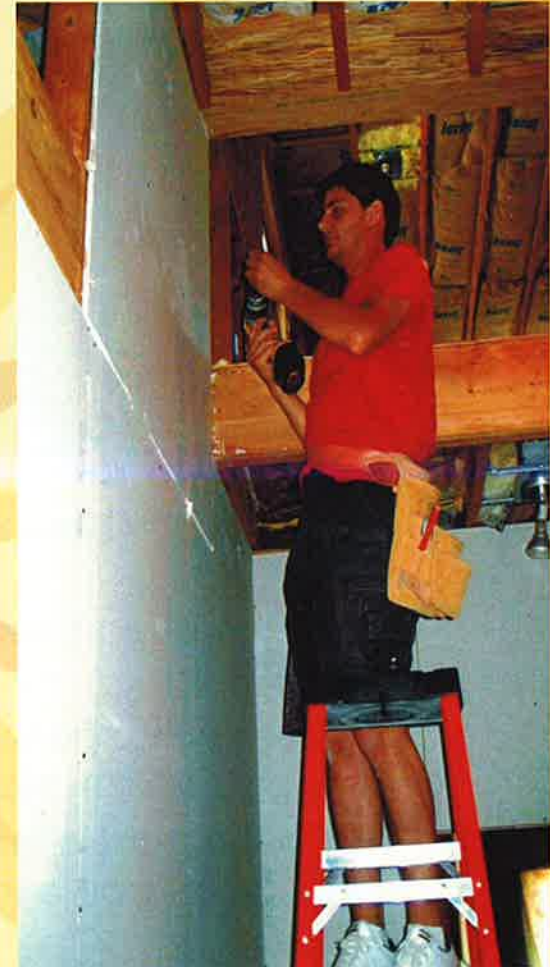
Brian hanging drywall at the shore house his parents are building.
